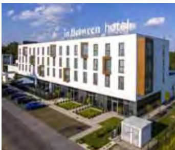
Hotel In Between, Jastków k. Lublina
